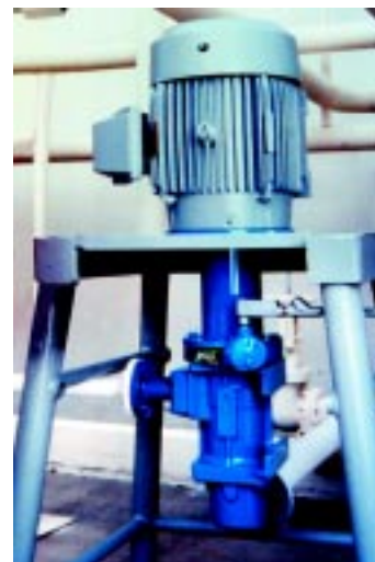
Vertical, Magnetic Drive 3D-250 pump on chemical service - Freeport, Texas, USA
