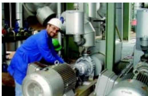
ALLHEAT® series pump in heat transfer fluid service - Germany
